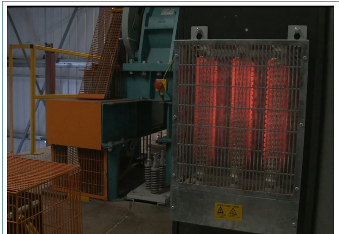
Before: Excess Energy Lost Through Braking Resistors
